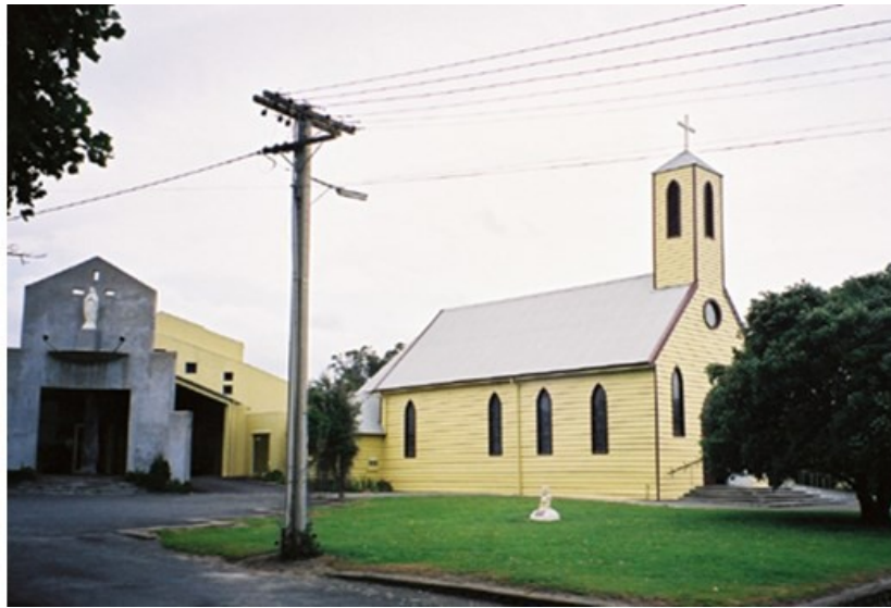
St Mary's, Pukekarakā. Copyright: NZ Historic Places Trust. Photograph by Helen McCracken
